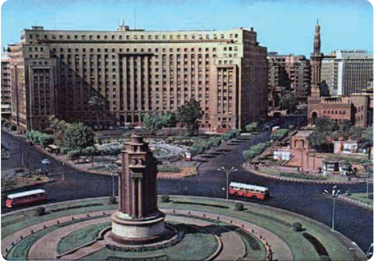
A photograph of the granite pedestal of the statue of Khedive Isma'il in Cairo showing the relation of the pedestal to Tahrir Square and its famous buildings. It was taken in the late sixties.
